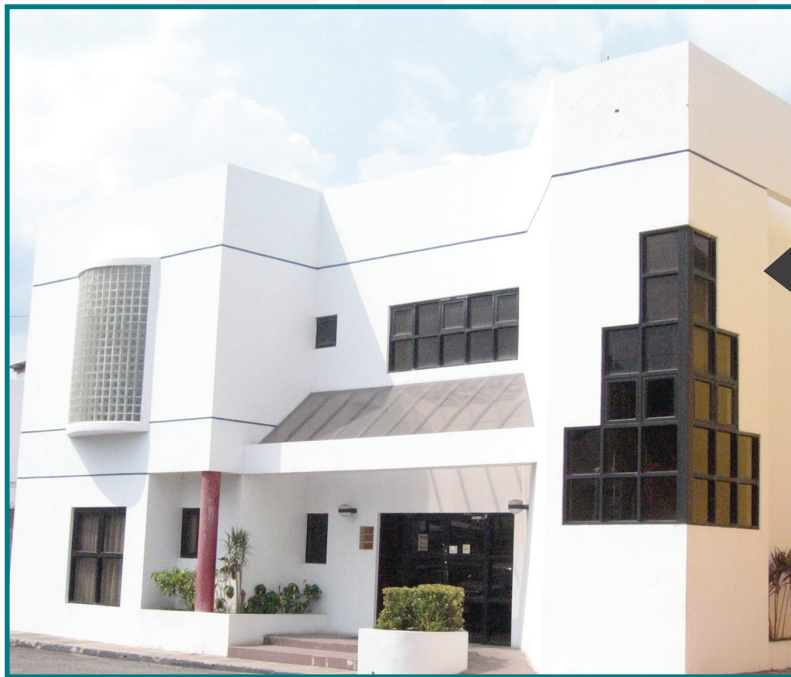
Red Hills Road Office
